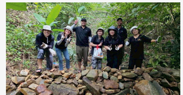
Construction of control dams for sustainable water catchment areas, Thailand.
